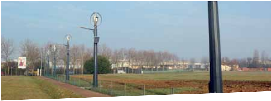
Stand-alone lighting installed at Orlytech
