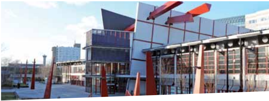
The Aeronef building houses Aeropole and Datagora.
