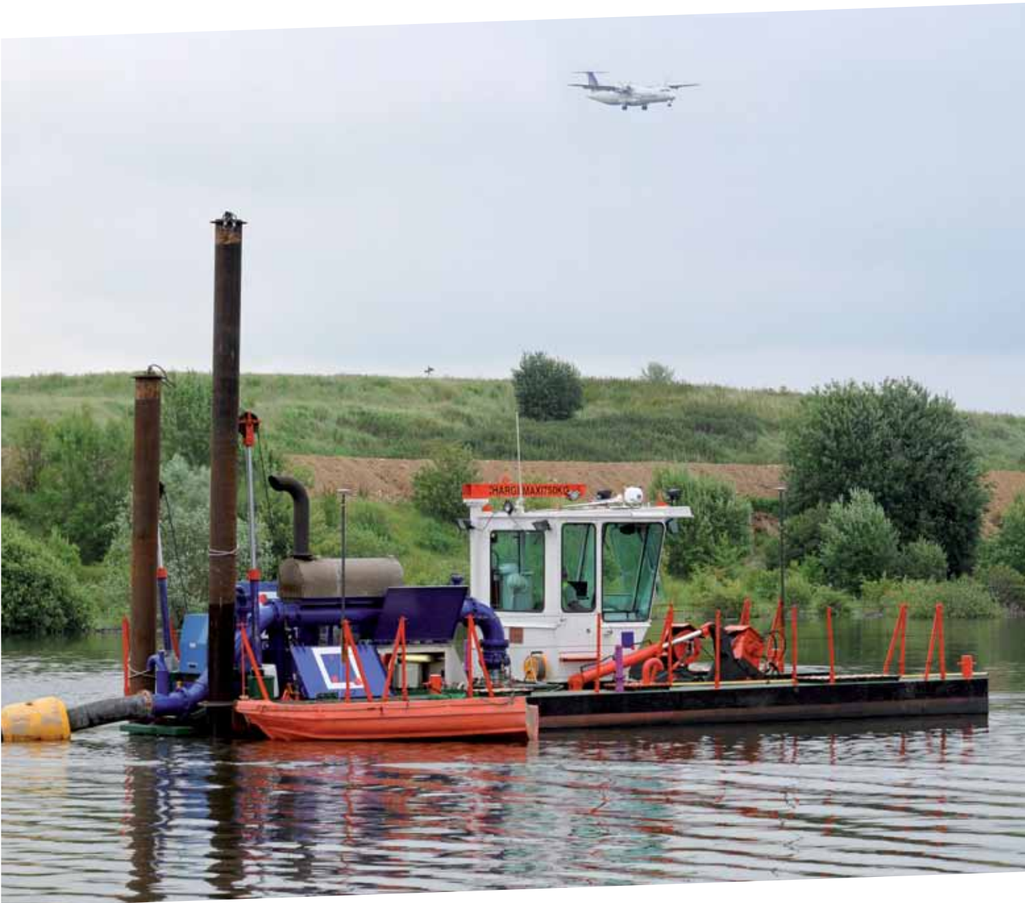
Cleaning the rainwater retention pond at Paris-Charles de Gaulle
