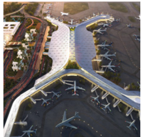
The new terminal at the Haikou Meilan international airport
