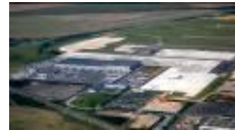
Fedex logistic centre phase 1.2
