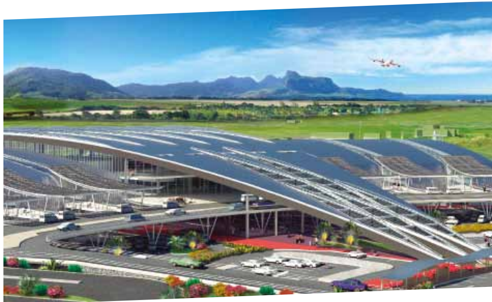
The new terminal designed by ADPI under construction on Mauritius, to be opened and operated by Aéroports de Paris Management.
