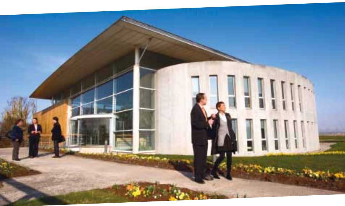
The Environment and Sustainable Development Centre at Paris-Orly.
