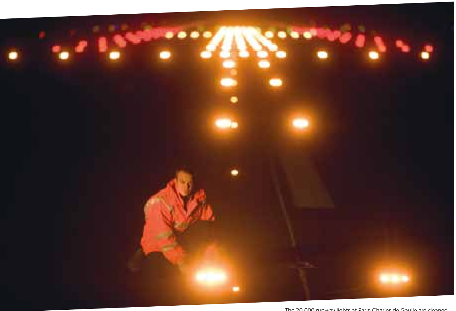
The 20,000 runway lights at Paris-Charles de Gaulle are cleaned by dry ice blasting with no rinsing and no residue.
