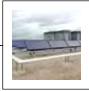
Solar panels on the roof of the Altaï building
