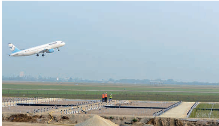
Since 2013, a filter marsh planted with reeds has contributed to lowering amounts of pollution in part of the stormwater runoff at Paris-Orly.
