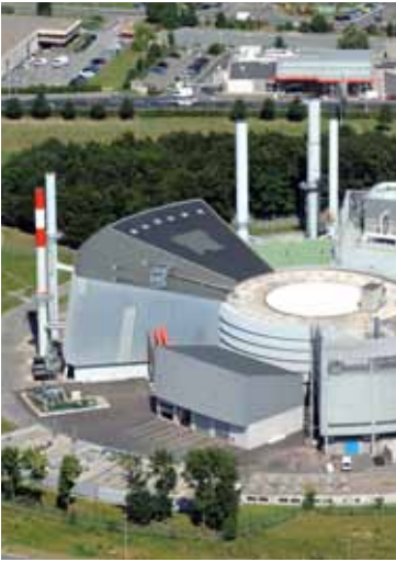
Two wood-fired boilers at Paris-Charles de Gaulle provide 25% of the heating needed at the airport without releasing fossil-fuel CO 2 emissions.
