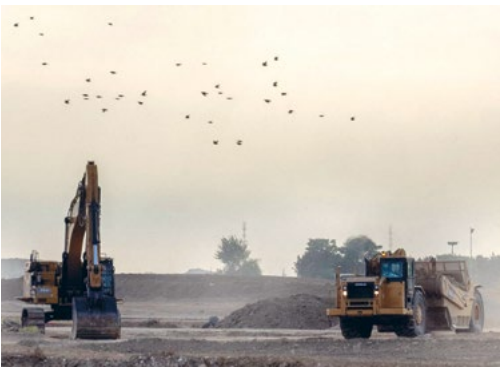
2 The complete renovation of runway 3 at Orly, a highly technical project, was completed on deadline - to the day.
