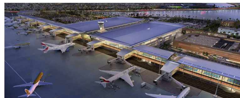
New terminal at Bahrain Airport ©ADP Ingénierie
