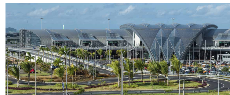
New terminal at Mauritius Airport ©A.Leduc - ATOL
