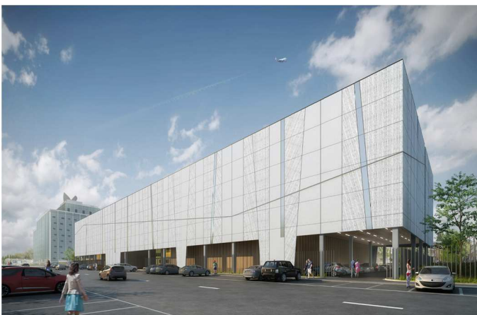
West view of the future storage and conservation centre for artworks at Paris-Le Bourget Airport © GBL Architectes
