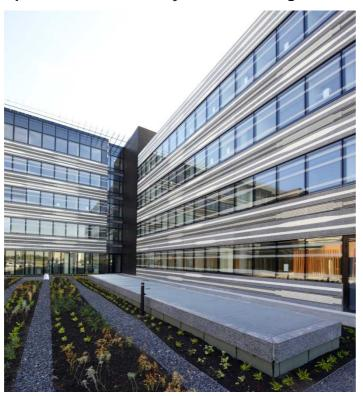
Designed by architectural firm Art & Build, Altaï has a U-shaped construction standing four storeys tall with two additional underground levels. The façade is composed of concrete, polished to a perfectly smooth and featuring multiple encrusted colours, and screen-printed glass.
