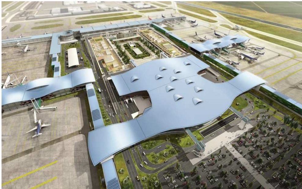
Aerial view of the future international terminal at Santiago
